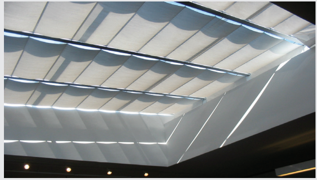
SkyLighter® shades, St. John's Bread and Life, Brooklyn, N.Y., Rogers Marvel Architects.
